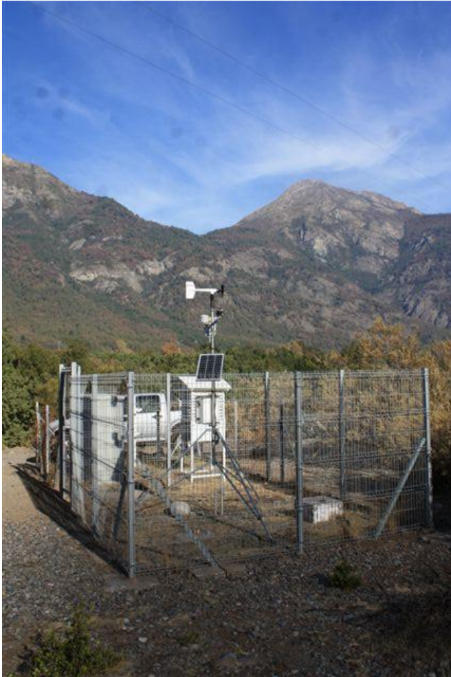
A private network installation (Speedwell, Chile)
